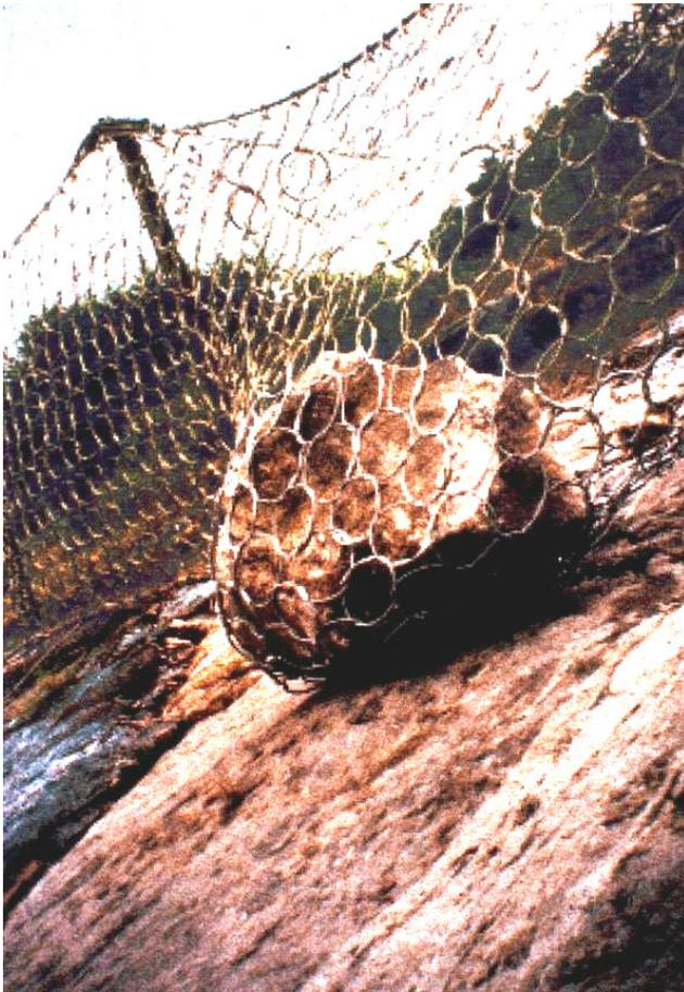
b: Geobruigg ring net shown restraining a boulder. These nets can be designed with energy absorbing capacities of up to 2500 kNm which is equivalent to a 6 tonne boulder moving at 20 m per second.
